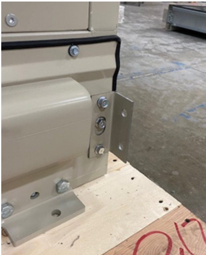
Figure 100: Lifting lugs located on base rail
