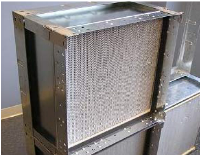
Figure 35: Properly Installed HEPA Filter
