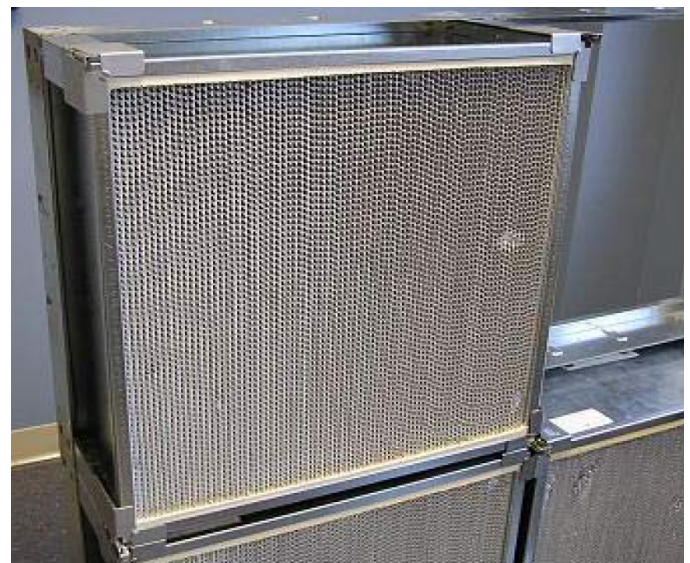
Figure 30: Properly Installed Filter Inside of the Frame
